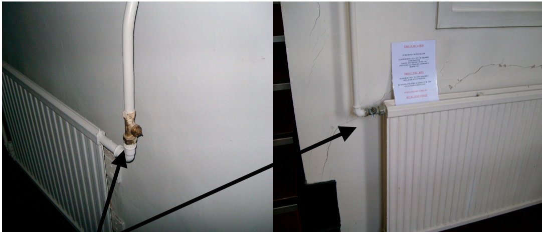
TRV's missing from radiators
